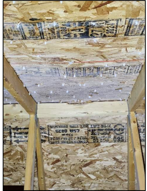
19. Water damage
