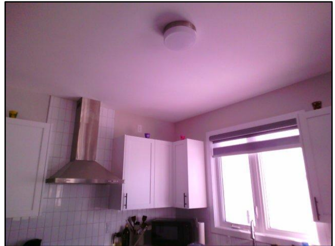
47. No elevated moisture found with meter
