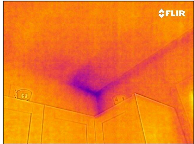
45. No elevated moisture found with meter
