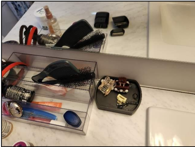
35. Caulking missing or ineffective
