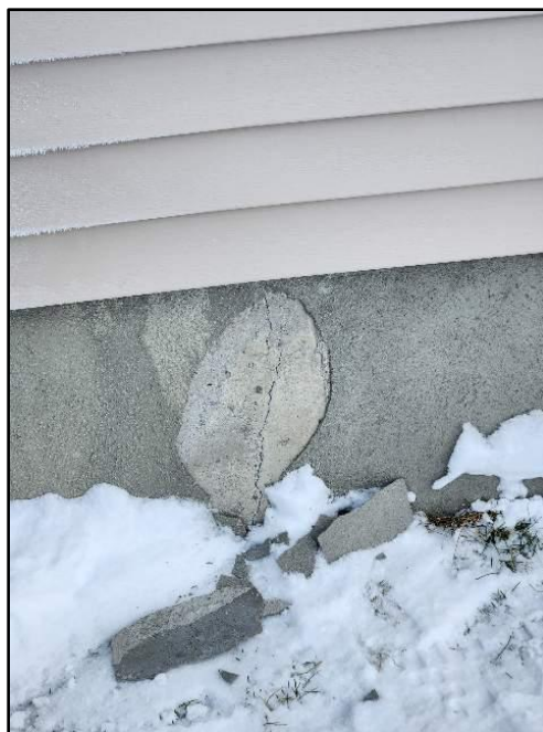
62. 1.10 Cast-in-place concrete foundation w
