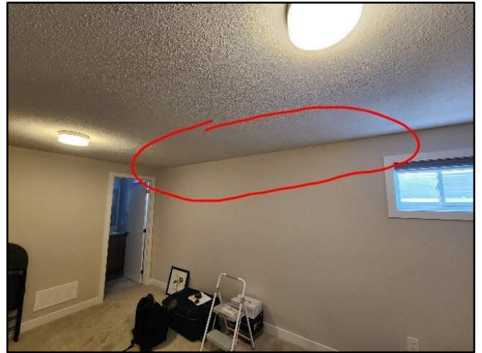
39. No elevated moisture found with meter
