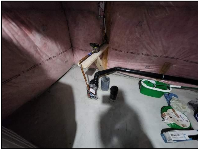
50. No elevated moisture found with meter
