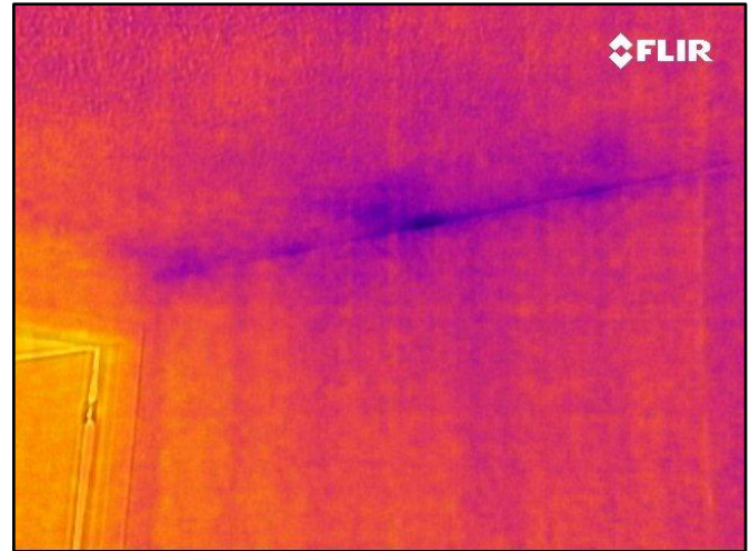
43. No elevated moisture found with meter
