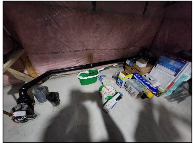
51. No elevated moisture found with meter
