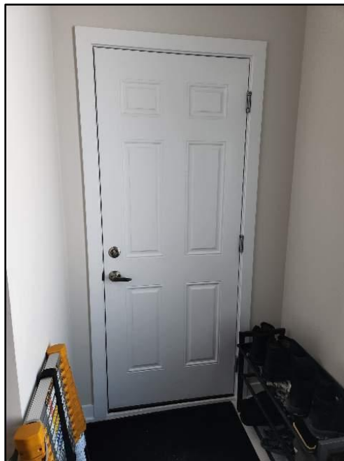
92. Garage man-door auto-closer not function
