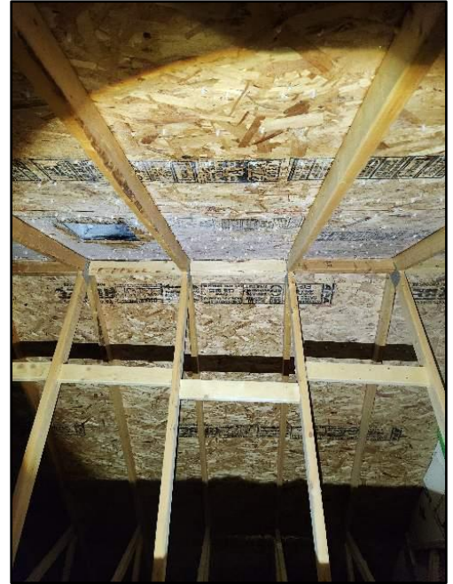
23. Water damage
