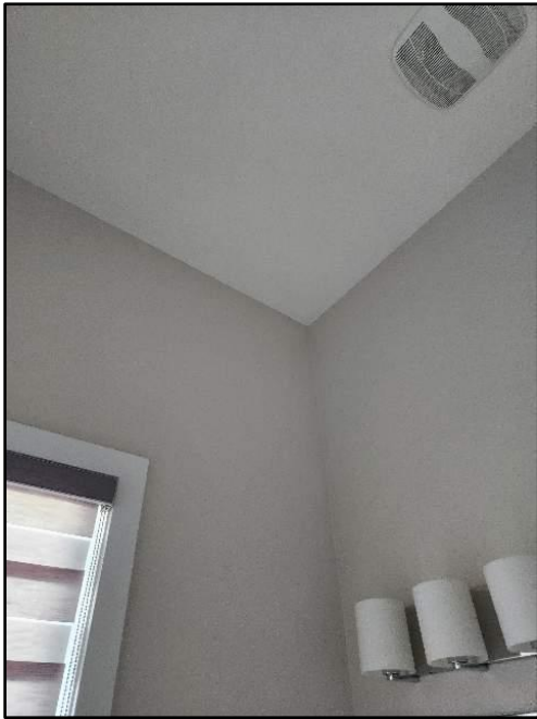
44. No elevated moisture found with meter
