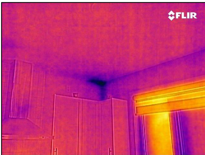
48. No elevated moisture found with meter
