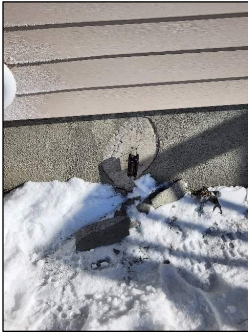
60. 1.10 Cast-in-place concrete foundation w
