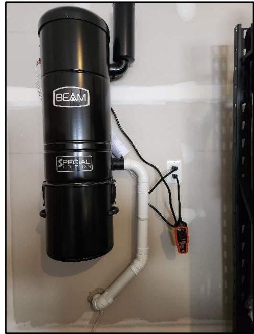
70. 7.1 Fuses blow or circuit breakers trip.
