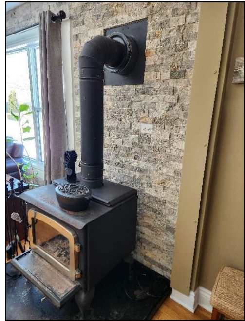
58. Side or back wall - combustible clearanc
