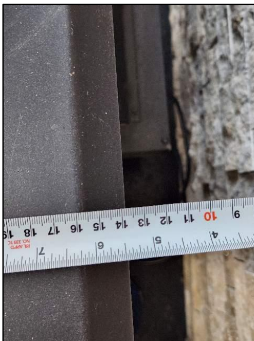
59. Side or back wall - combustible clearanc
