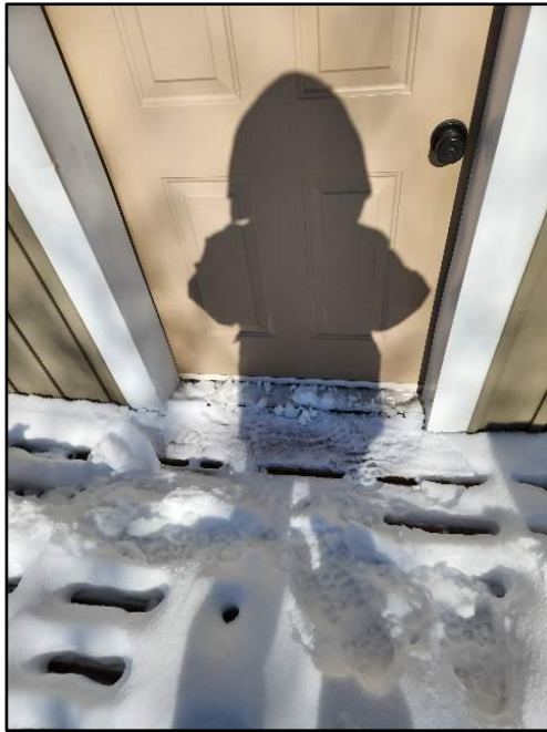
18. No step up into building
